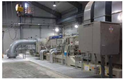
EMD Compressor Train utilizing Voith Hydrodynamic Gearbox
